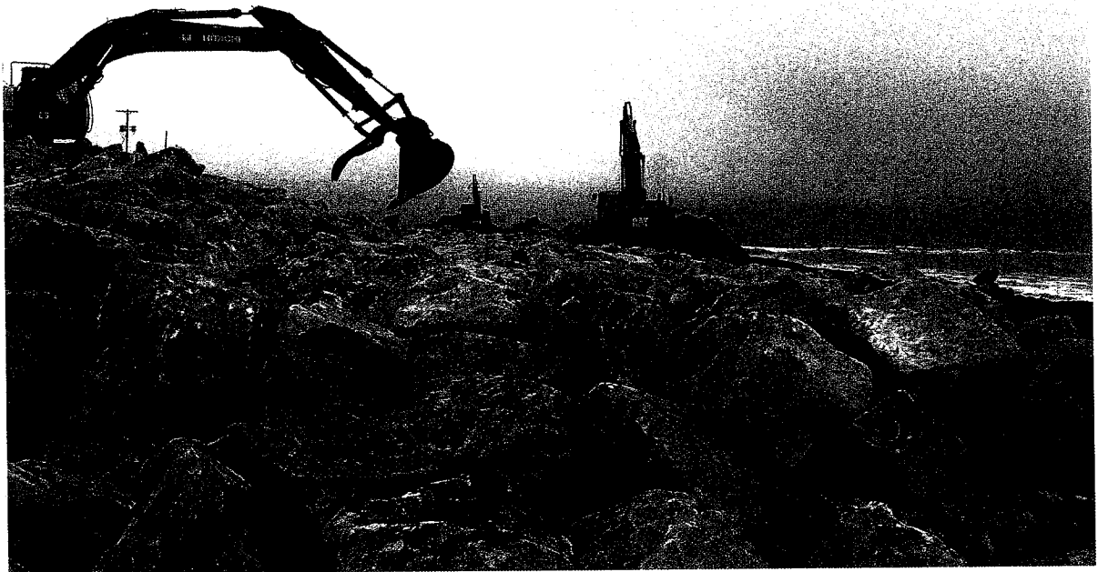
Constructing a seawall at Kivalina in Northwest Alaska, an Inupiat Eskimo community on a barrier reef between the Chukchi Sea and Kivalina River which has been hard hit by continuous erosion. PHOTO COURTESY OF BRICE INC.
